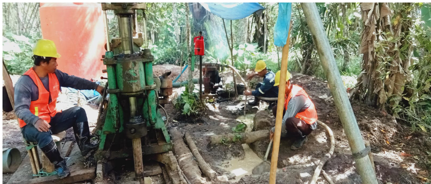
Proses pengeboran di Kab. Ngada. Kedalamannya mencapai 105 meter dan dapat menghasilkan hingga 100 kubik air per hari. The drilling process in Ngada District. Its depth reaches 105 meters, producing up to 100 cubic meters of water daily.
